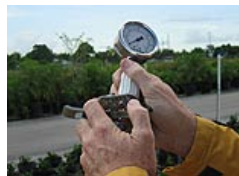
Figure 8. Mobile Irrigation Lab: Measuring sprinkler pressure (Source: SWFWMD, https://www.swfwmd.state.fl.us/agriculture/mobile.html )
